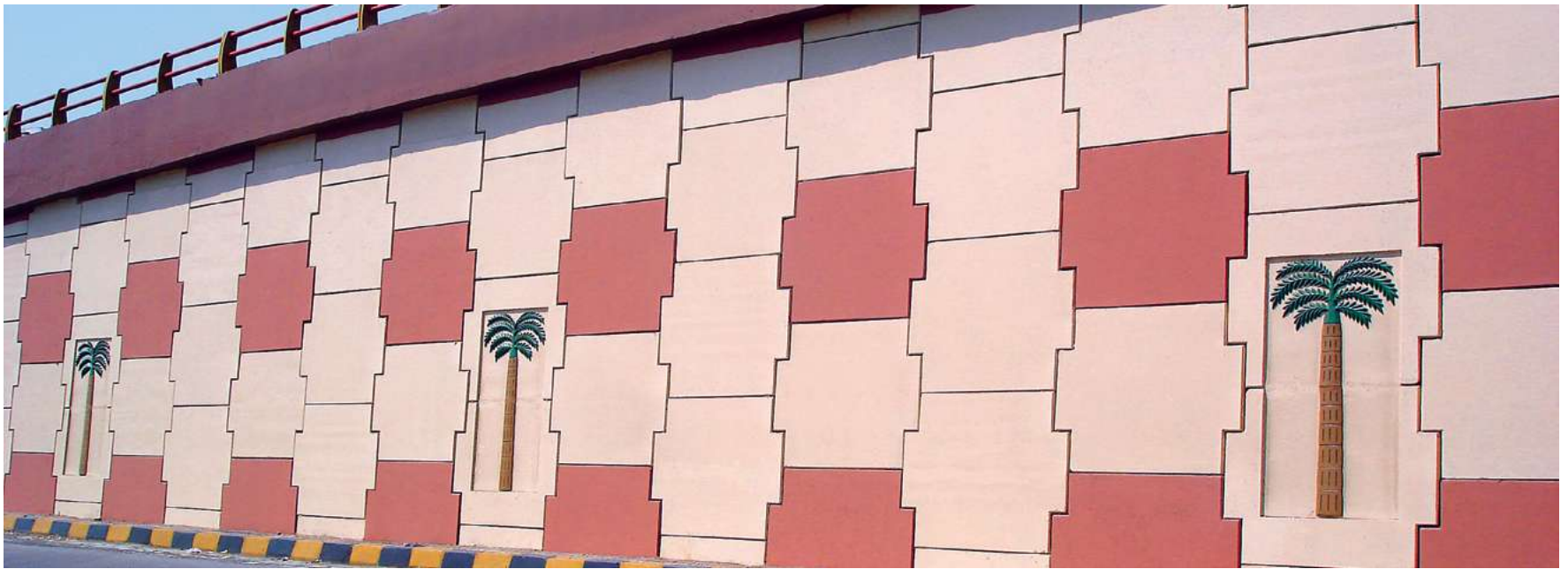
Navghar Flyover, Mumbai International Airport Mumbai, India ►
