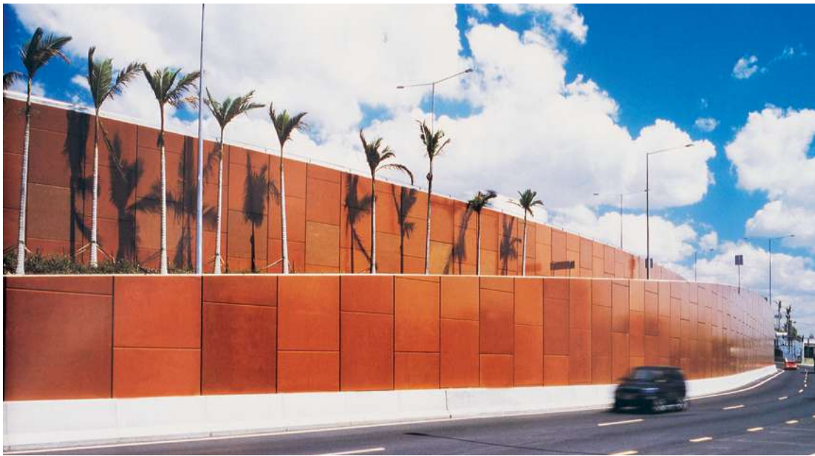
Inner City Bypass Brisbane, Queensland, Australia ►
