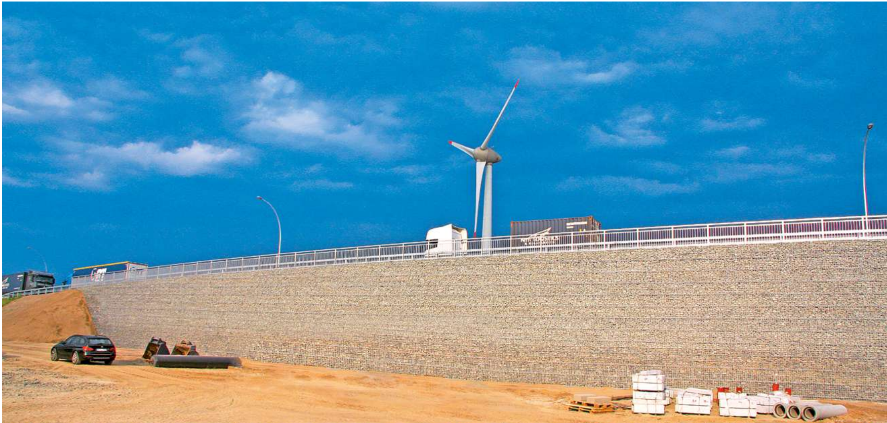
Retaining Walls in Altenwerder
