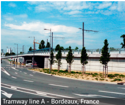
Tramway line A – Bordeaux, France
