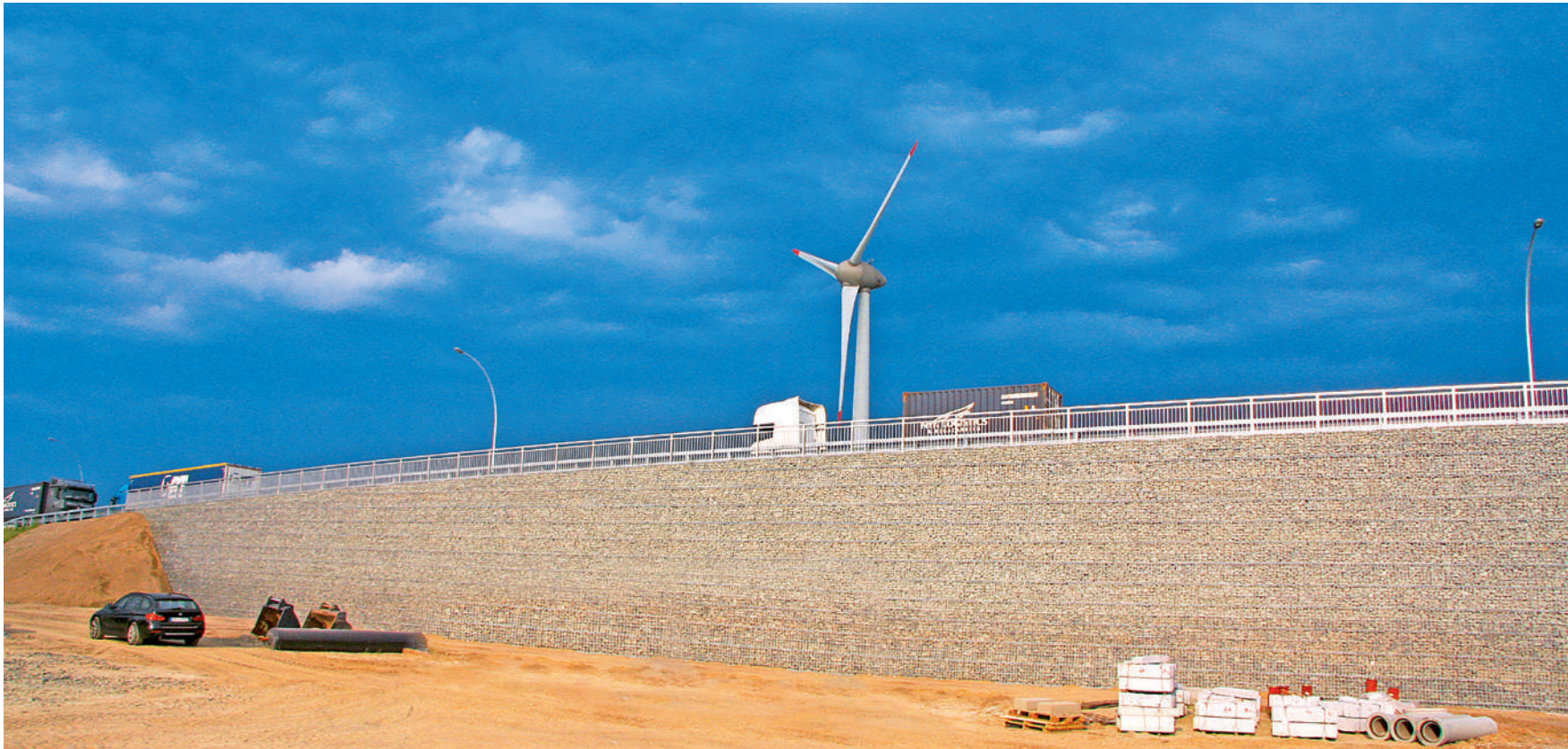
Retaining Walls in Altenwerder
