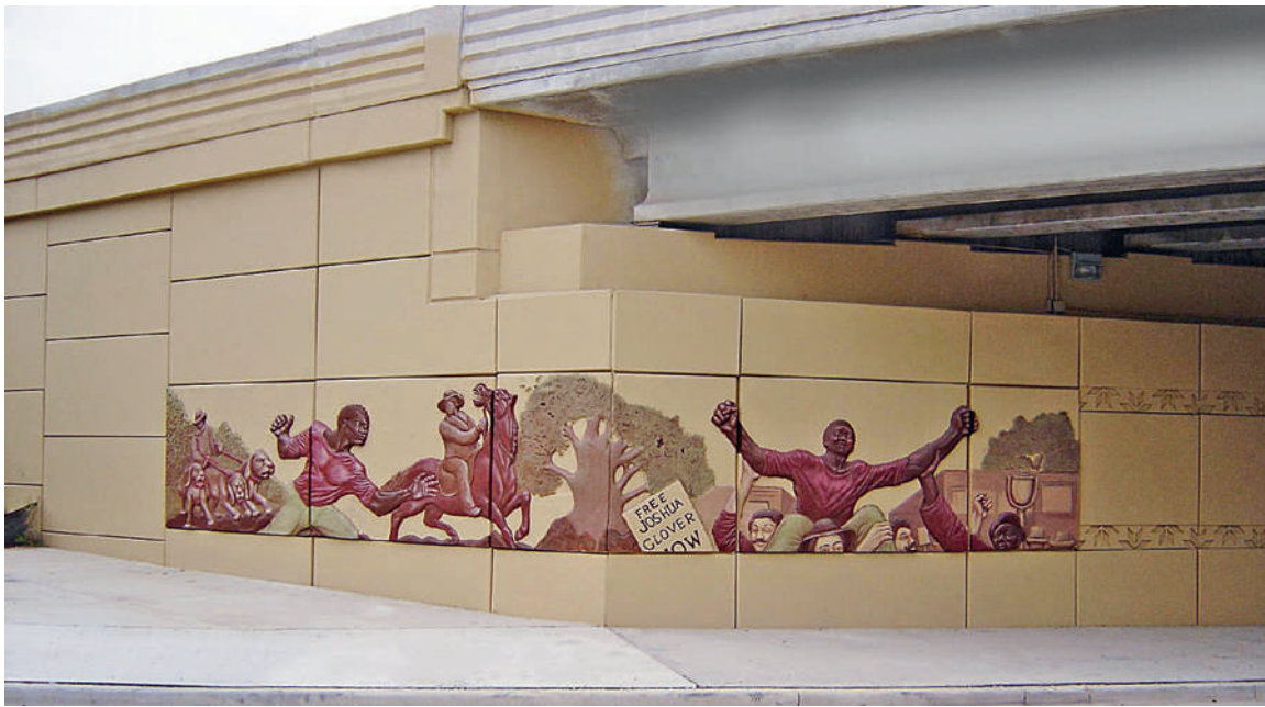
Marquette Interchange Milwaukee, Wisconsin, USA ►
