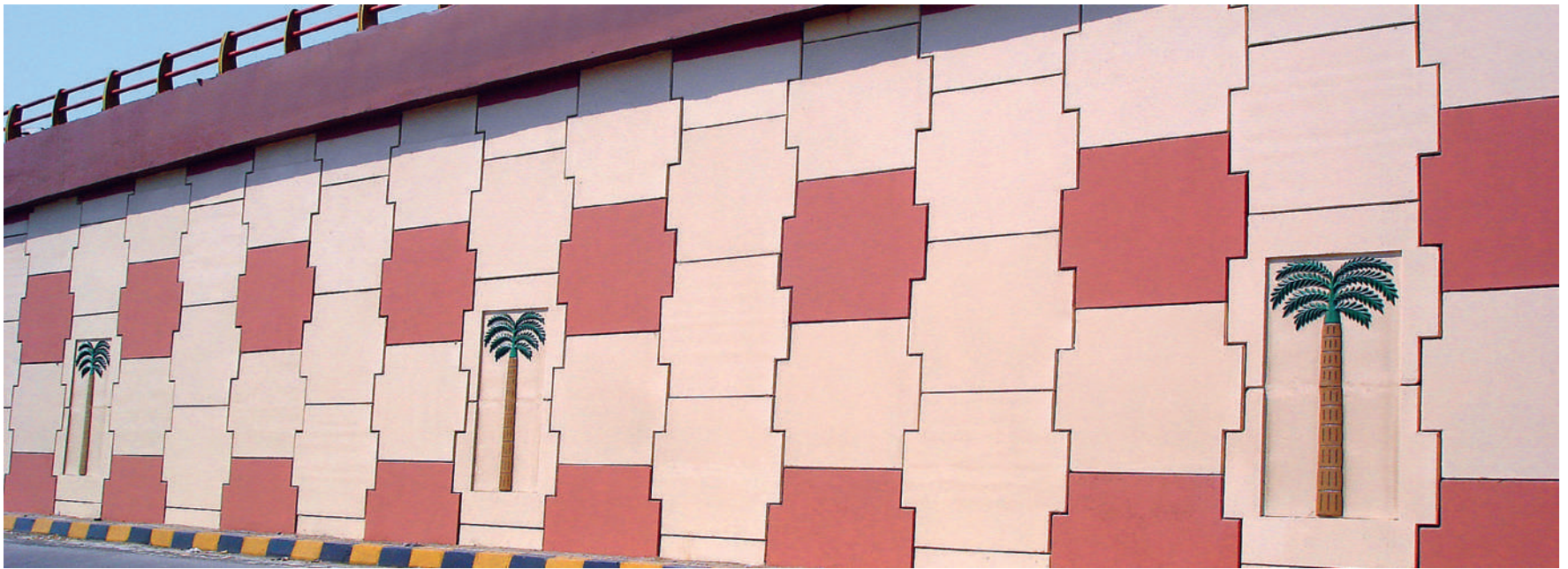
Navghar Flyover, Mumbai International Airport Mumbai, India ►
